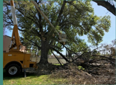
Removing a downed branch at Sterling Ave.
